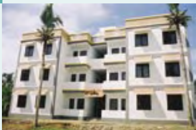
Apartments in Thekkawatta, Kalutara, Sri Lanka
